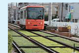
Rail track greening
